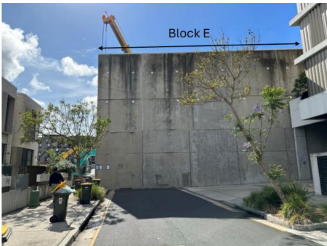
Figure 3: Site viewed from Metters Street looking east
