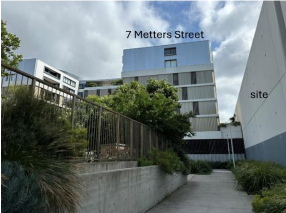
Figure 6: Pedestrian link between subject site and 74 Macdonald Street looking north to rear of 7 Metters Street
